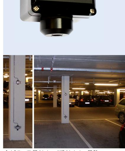
Installation with CO detector and HC detector type GP-SA.
